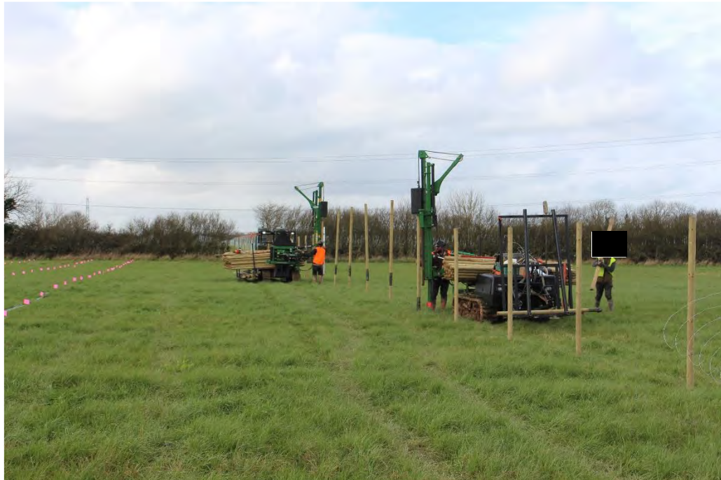
Plate 6: Establishment of Site fencing
