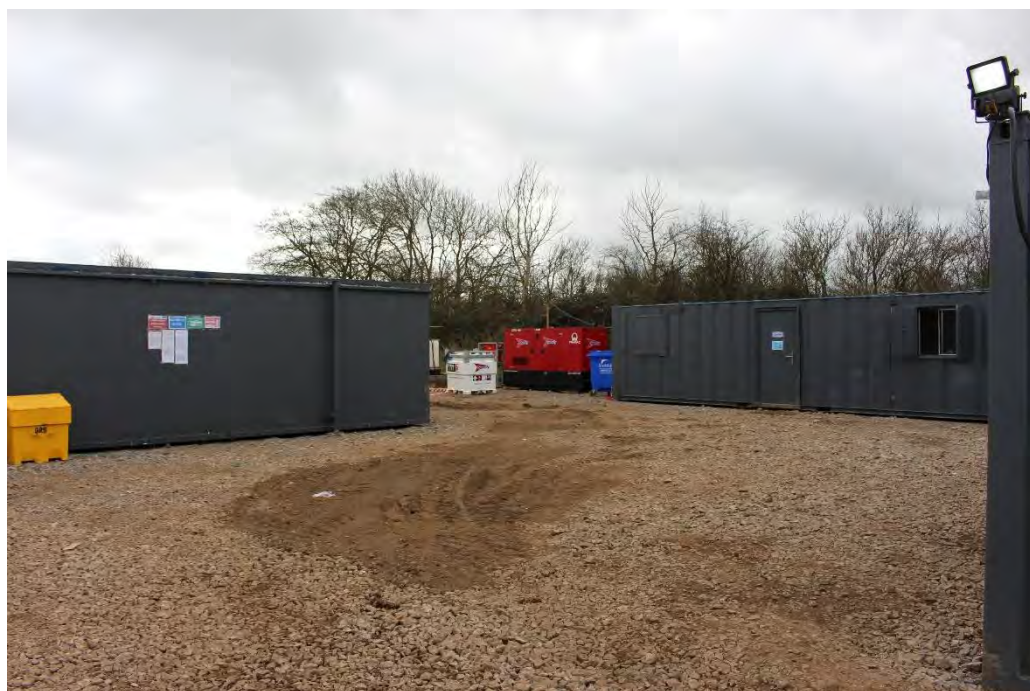
Plate 7: Establishment of the temporary construction compound(s)
